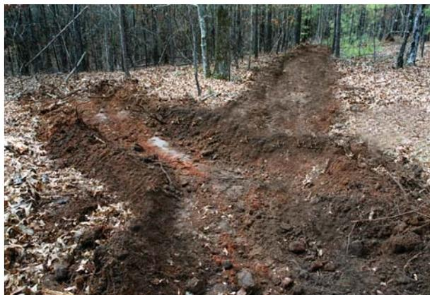
An appropriate water diversion moves water away from the main firebreak and into a stable vegetated area.
