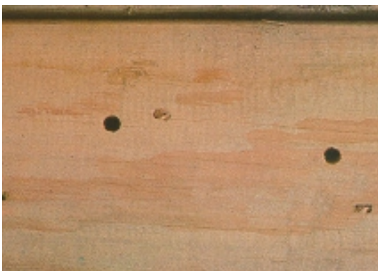
Fig. 15. Carpenter bee holes can be distinguished from other insect holes by their size and rounded shape. (GFC Photo)
