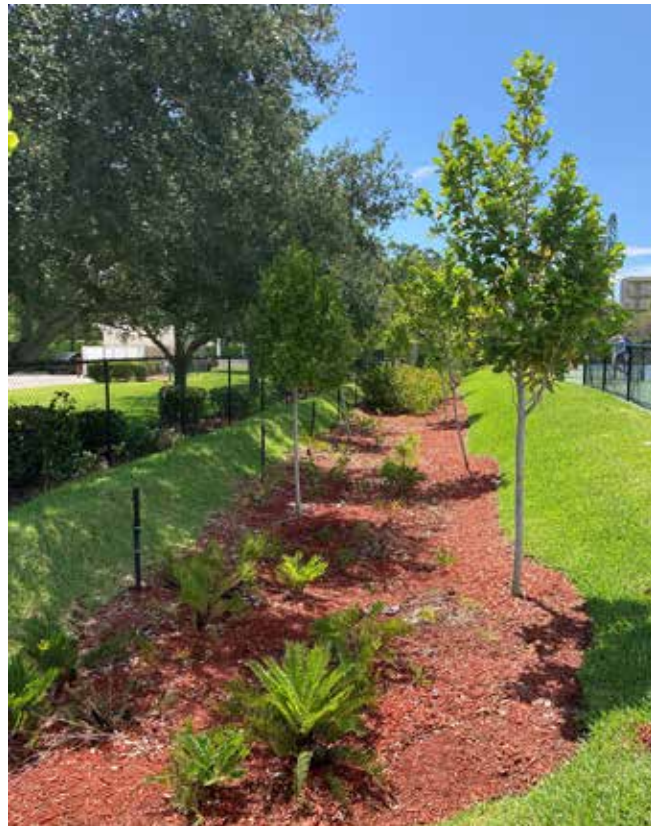
These trees planted in a bioswale will help to soak up more stormwater and are also infrastructure for this Florida city.
