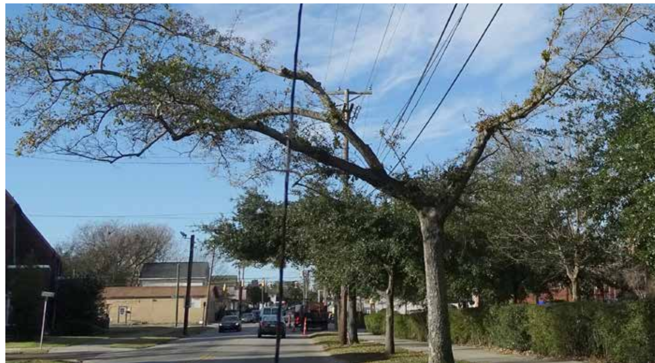
Avoid planting large trees under power lines. Smaller trees, such as crab apples ( Malus ) or crepe myrtles ( Lagerstroemia ), can be planted and not interfere with overhead wires.
