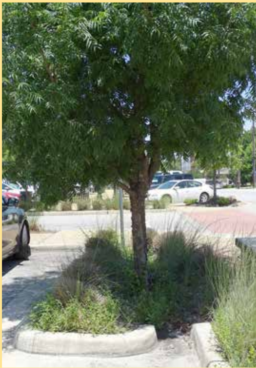
This tree in a bioswale is green infrastructure because it is part of a stormwater best management practice (BMP).
