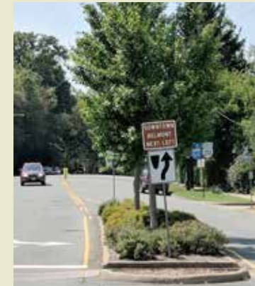
Streets were narrowed with new tree islands and bump outs with trees were added to sidewalks to shield pedestrians and slow traffic.
