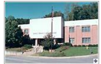
Banks County Courthouse
