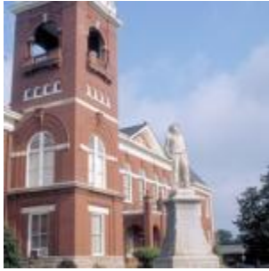
Butts County Courthouse
