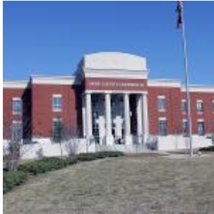
Crisp County Courthouse
