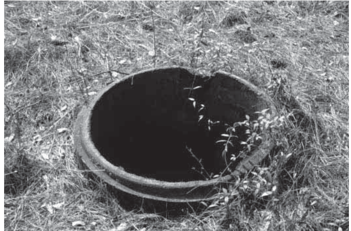
Figure 229 - Abandoned, uncovered water well
