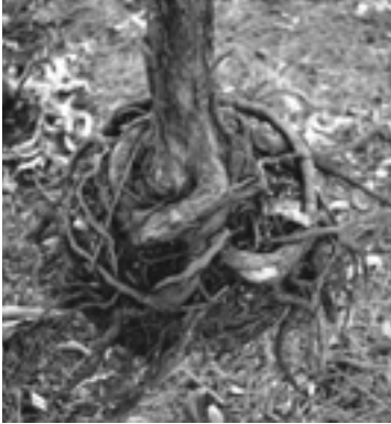
Poor nursery practices that produce girdling roots will cause early tree decline and death.
