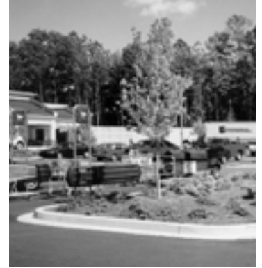
18'x36' tree planting island in a new parking lot provides sufficient prepared soil to establish two trees. However, additional space under the asphalt must be found for long-term tree growth.
