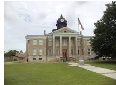
Irwin County Courthouse
