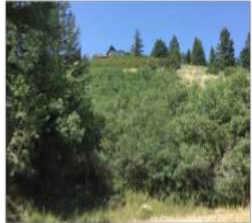
Homes built mid-slope and at the top of steep slopes and within ravines and draws are at greater risk of convective heat from wildfires. A wildfire could rapidly spread up this steep slope and threaten the home above. Photo credit: SafeScapes, LLC
