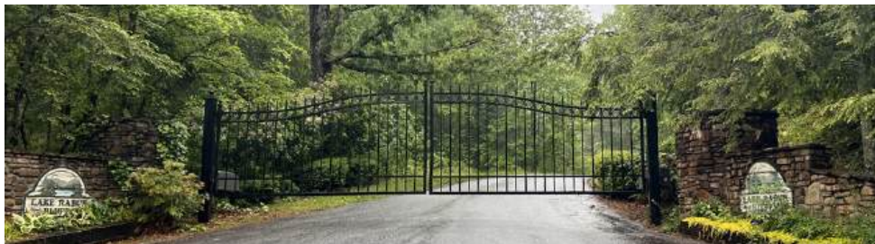
Locked gates can slow down firefighting efforts Photo Credit: SafeScapes, LLC
