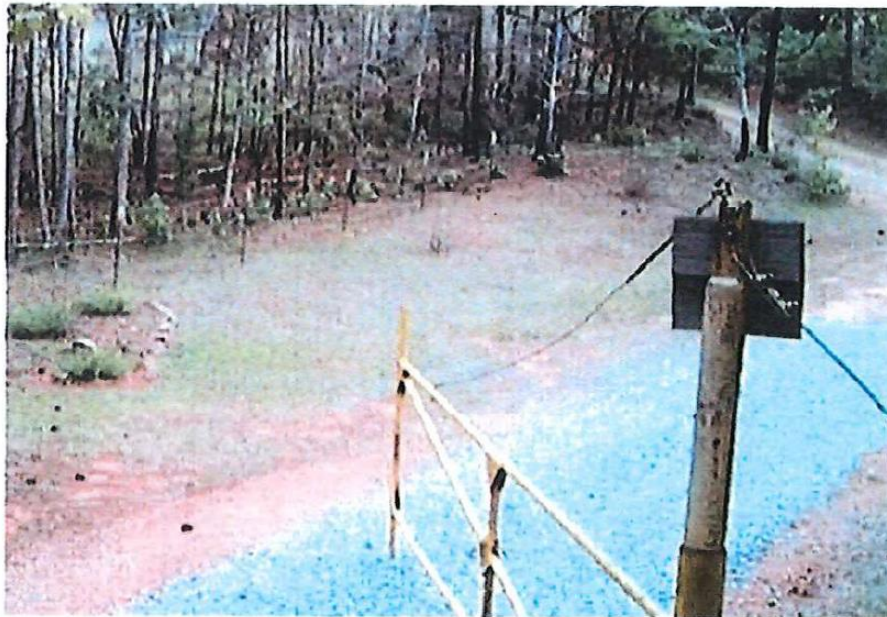
Picture 3 – showing gravel applied in high-traffic and sloped areas
