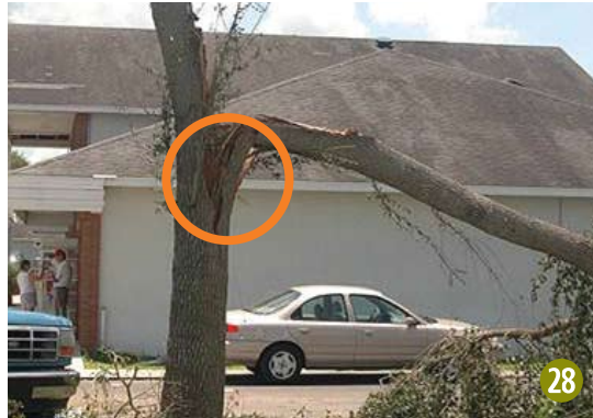
Figure 28 This tree should be removed since its broken stem is very large and the trunk is cracked, as shown by the circle. If the tree were not cracked into the trunk, the broken limb could be carefully removed and the tree might be restorable.
