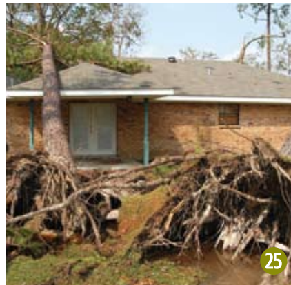
Figure 25 The high water table at this site restricted root depth and saturated soil allowed roots to slide in the soil, making these pines topple over during a hurricane.
