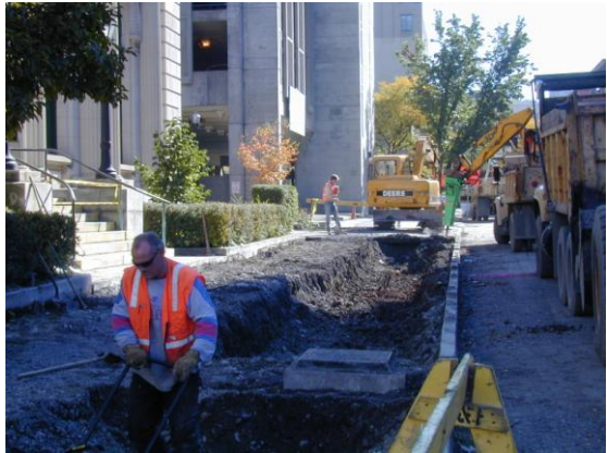
Typical structural soil streetscape installation (above). Trees growing in structural soil in high-use area (below). Photos courtesy of Dr. Nina Bassuk, Urban Horticulture Institute, Cornell University.
