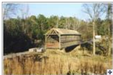
Auchumpkee Covered Bridge
