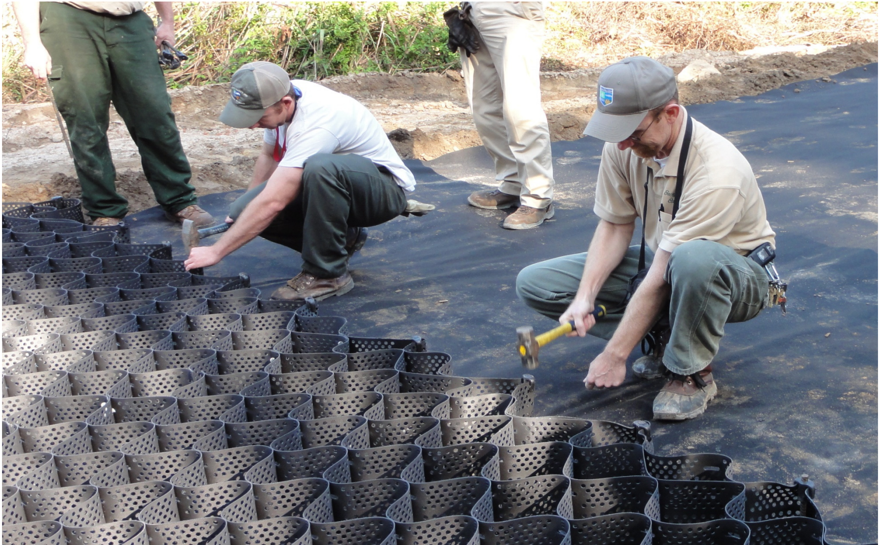
Securely staking down the end of the Geoweb.
