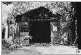
Cromer's Mill Covered Bridge
