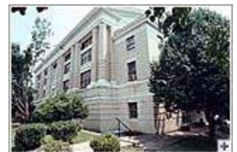
Walker County Courthouse
