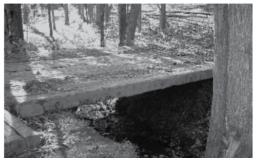
Portable timber bridge
