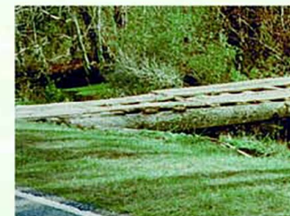
Pole bridges can be used for temporary stream crossings under certain conditions.
