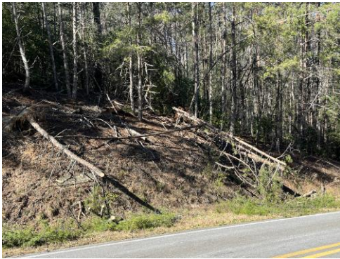
Figure 3: Light Damage in Habersham Co
